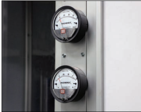
DUAL MAGNEHELIC® PRESSURE GAUGE Use for monitoring the positive or negative pressure differential between cleanroom spaces.
